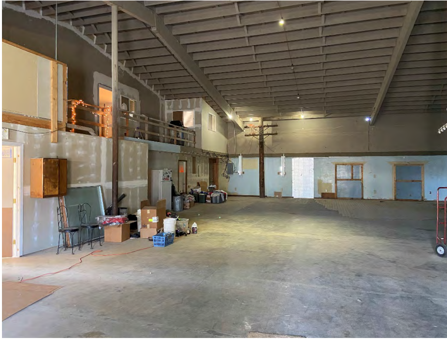
Photograph 7: View of the warehouse building interior.
