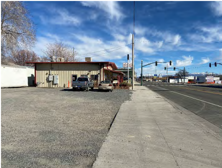
Photograph 18: View of the northeastern adjoining property, Cowpoke Café.
