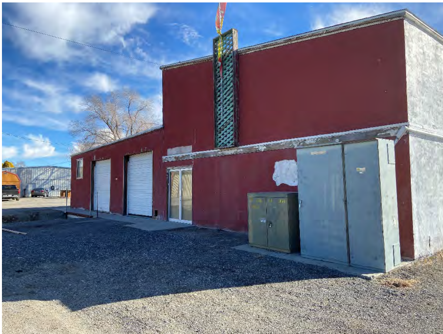
Photograph 2: View of the Property warehouse building, facing west with pad-mounted transformer.
