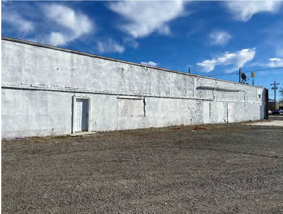
Photograph 1: View of the Property warehouse building, facing south.
