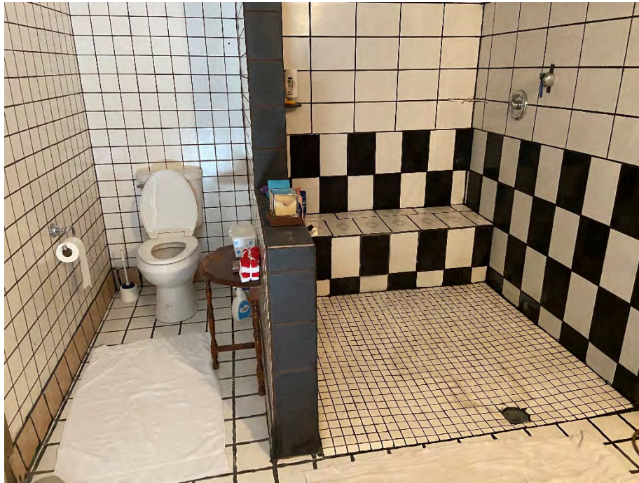
Photograph 11: View of restroom with floor drain inside the warehouse building.
