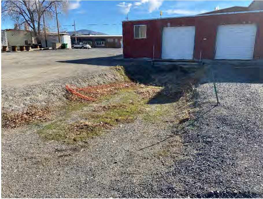
Photograph 3: View of the Property warehouse loading doors.
