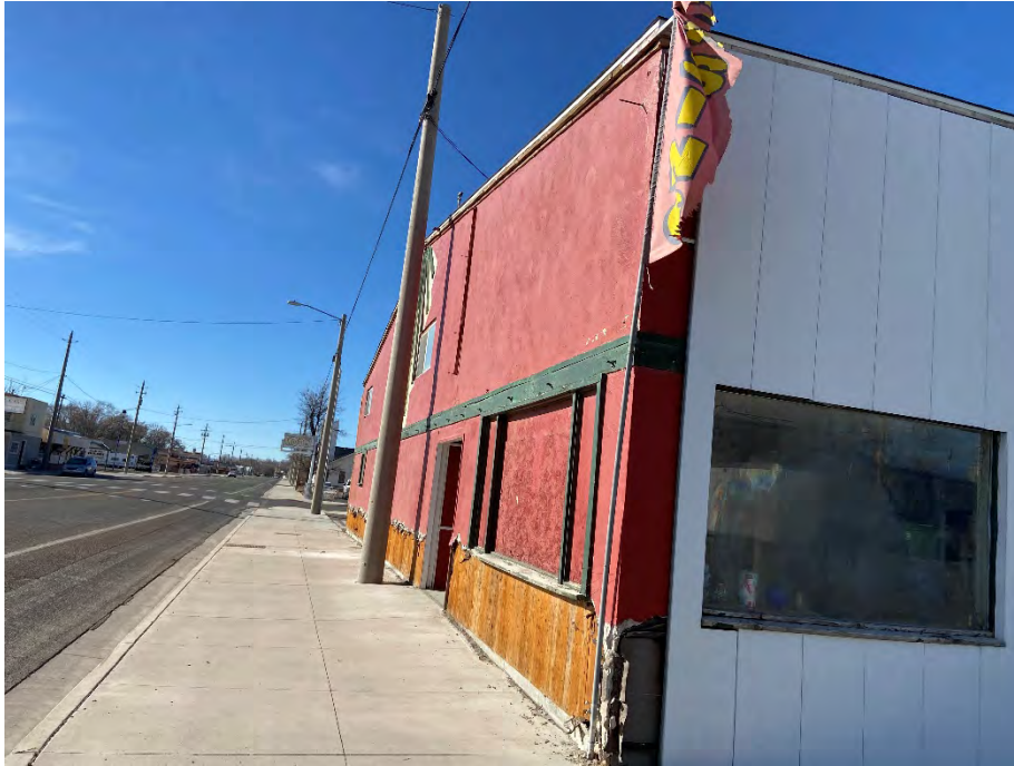
Photograph 5: View of the Property warehouse building, facing east.
