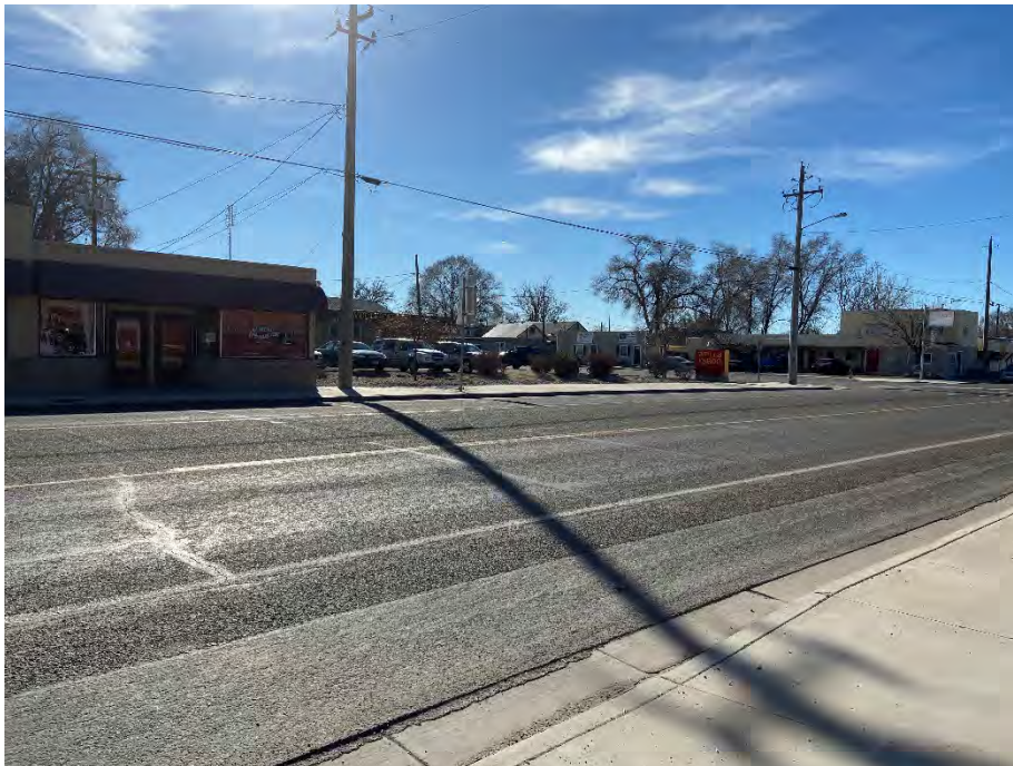
Photograph 20: View of the eastern adjoining property, Wells Fargo Bank.
