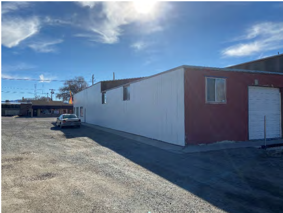
Photograph 4: View of the Property warehouse building, facing north.
