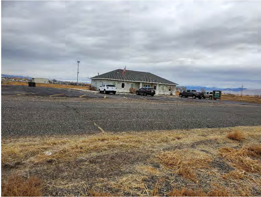
Photograph 13: View of northern adjoining property.
