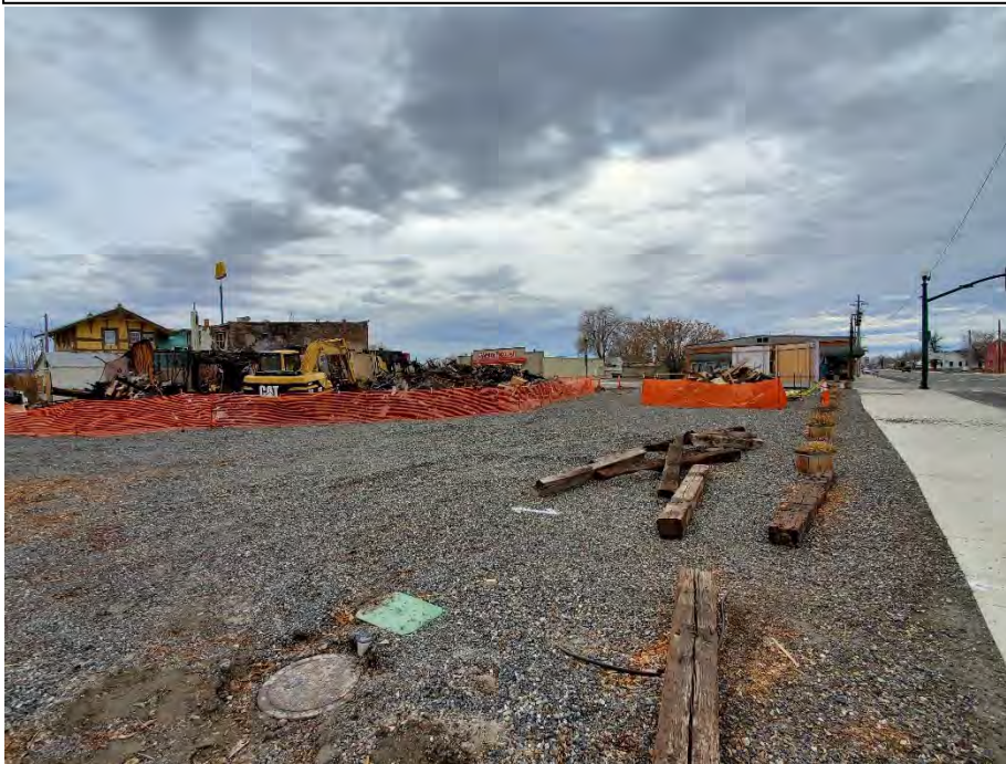
Photograph 10: View of the Property taken facing south.
