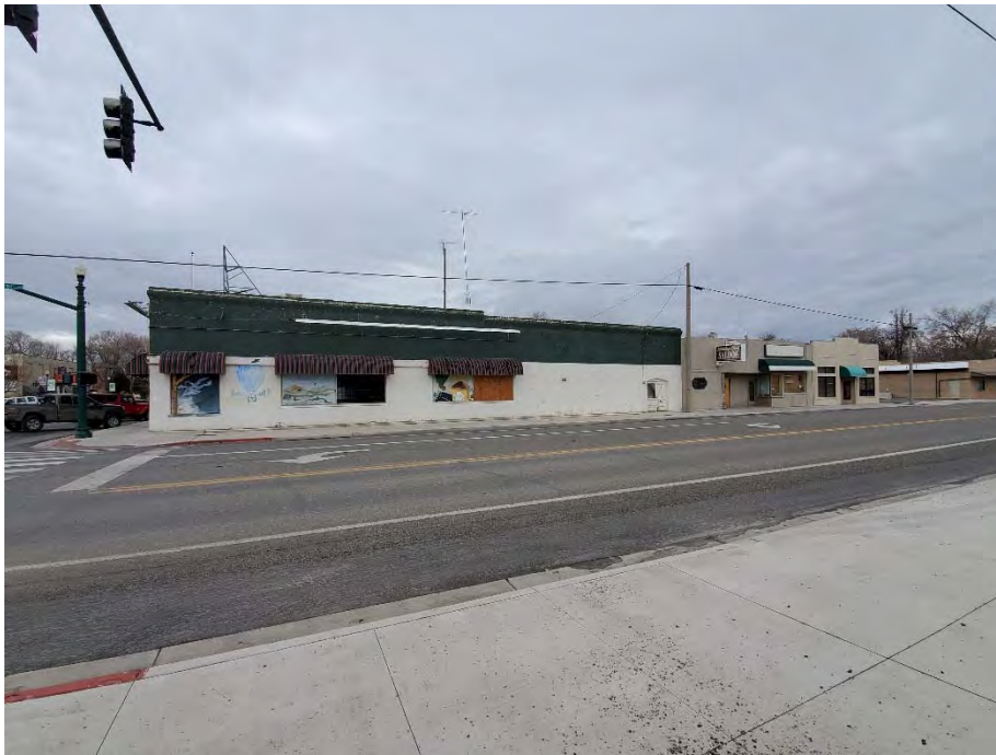
Photograph 8: View of northwestern adjoining property.
