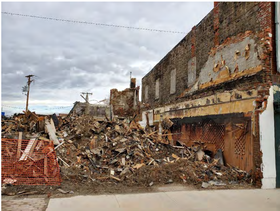
Photograph 2: View of 230 Main Street.
