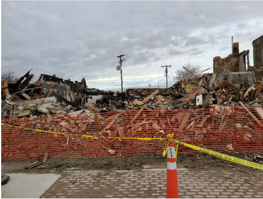
Photograph 3: View of southeastern adjoining property.
