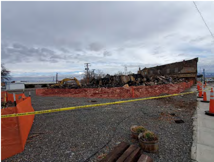
Photograph 6: View of remains of adjoining properties.
