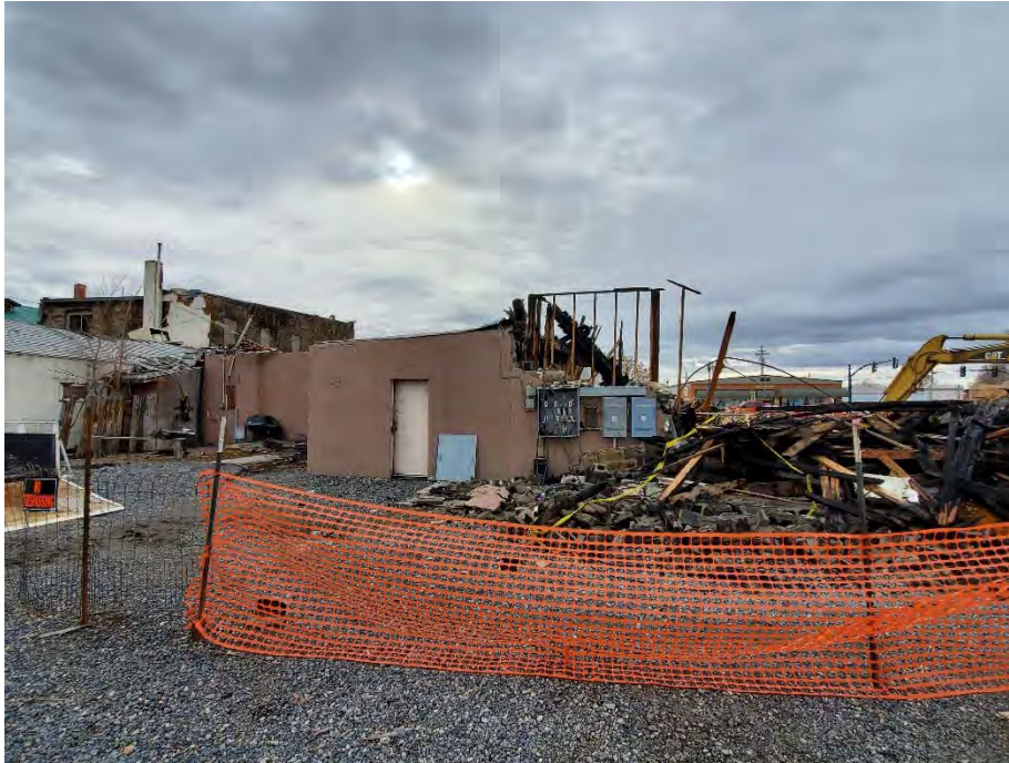
Photograph 11: Additional rear view of the Property.
