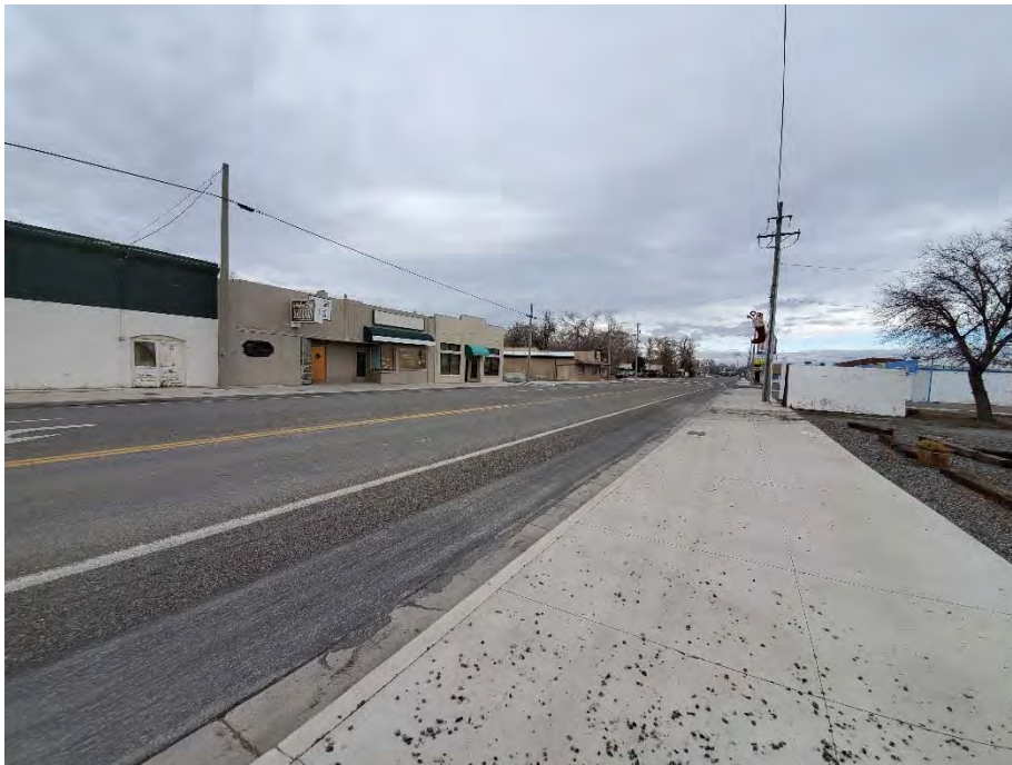
Photograph 16: View of Cornell Ave.
