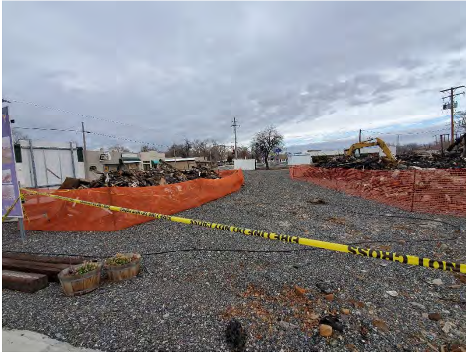
Photograph 3: View of northwestern adjoining property.
