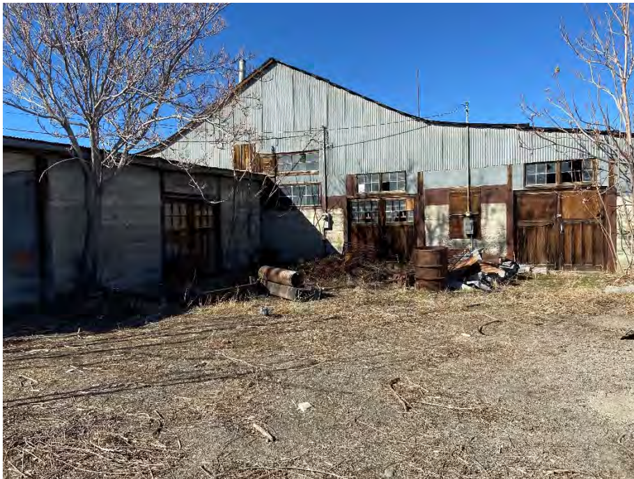
Photograph 6: View of western portion of the warehouse.
