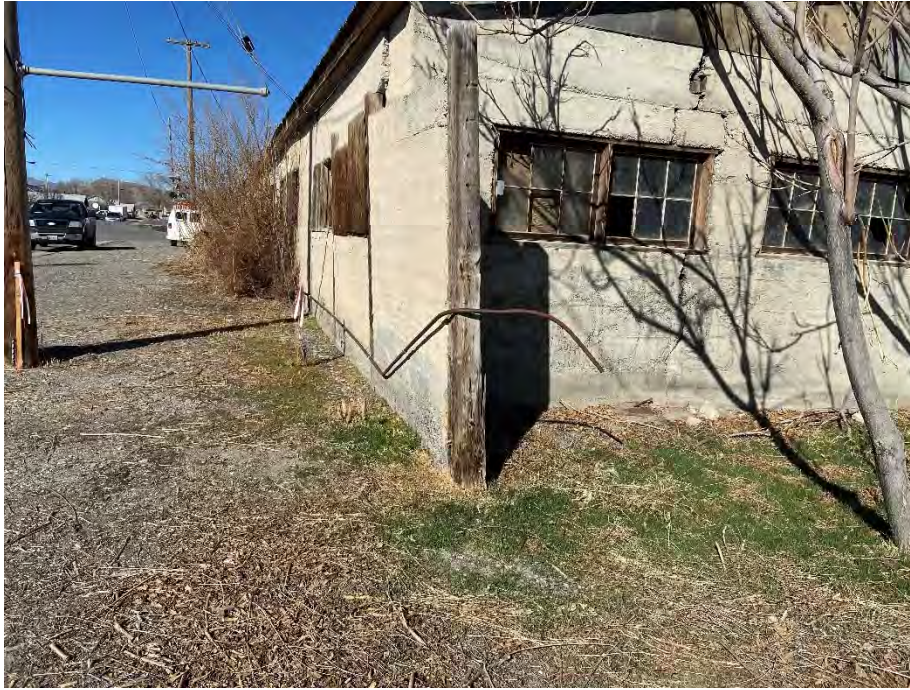
Photograph 11: View of the southern exterior of the warehouse.
