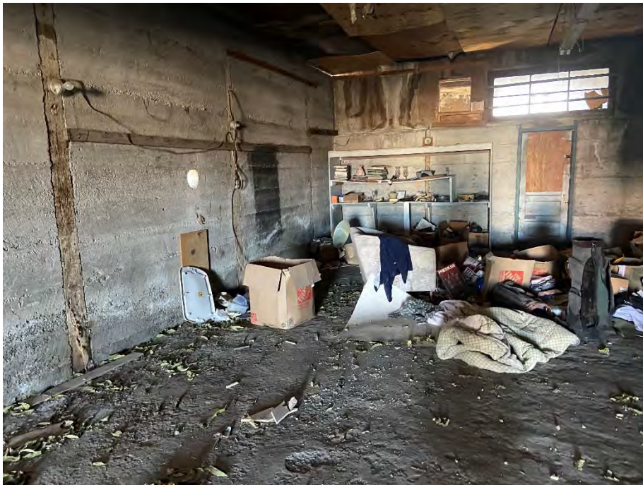
Photograph 28: View of storage in the warehouse area.
