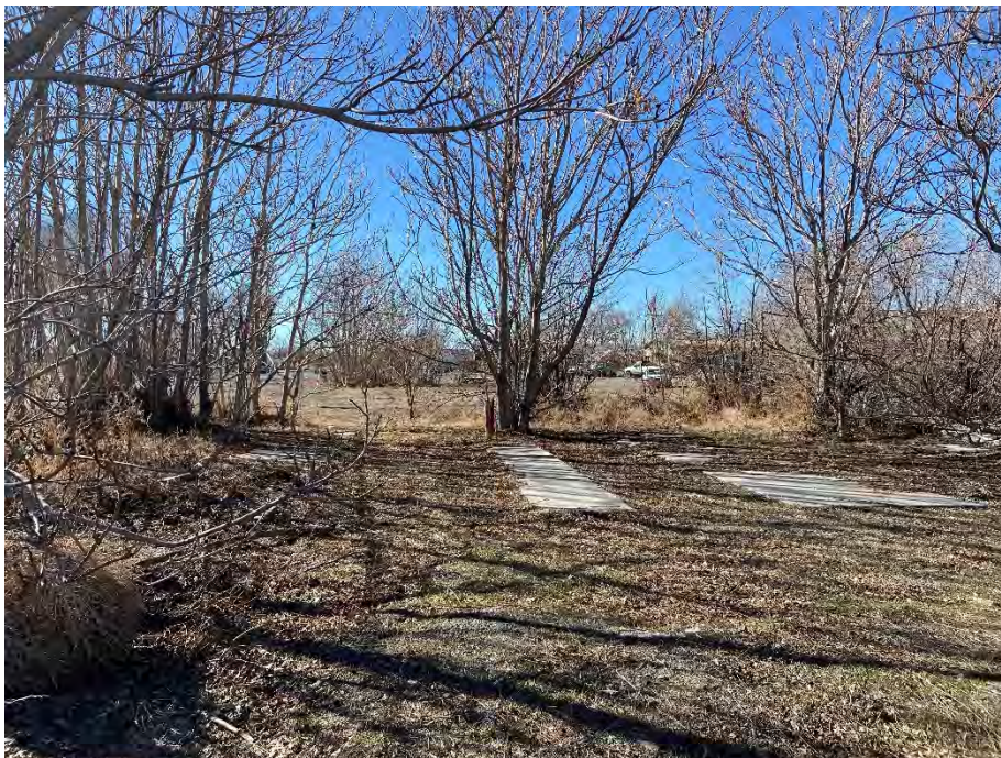
Photograph 14: Additional view of remnant building foundation on the northern portion of the Property.
