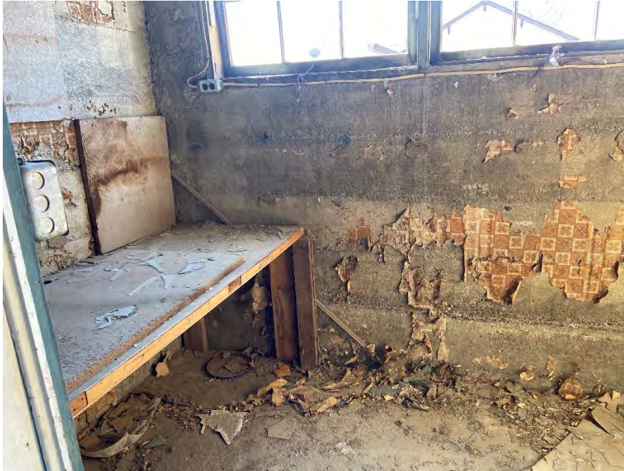
Photograph 27: View of previous office.
