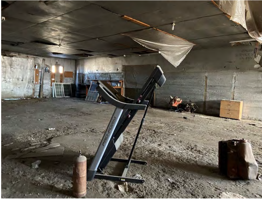
Photograph 29: View of another portion of the warehouse interior.
