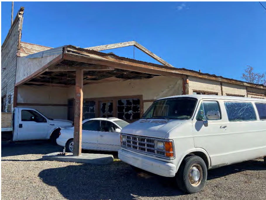
Photograph 2: View of fuel island on the southeast corner of the Property.
