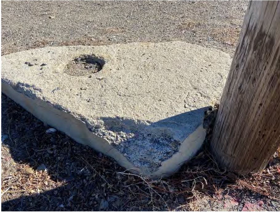
Photograph 3: View of potential former fill port.
