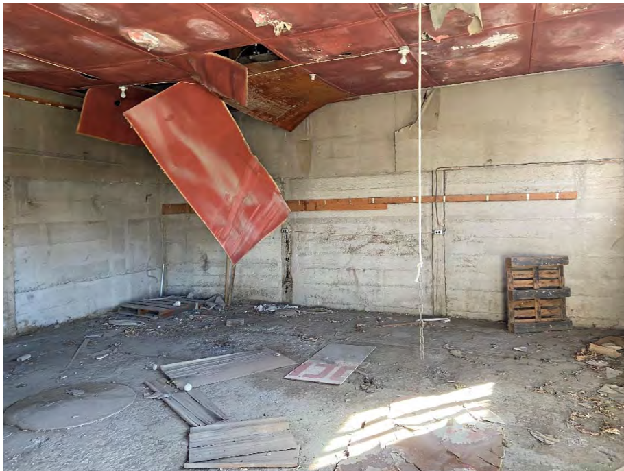
Photograph 26: View of general warehouse interior.
