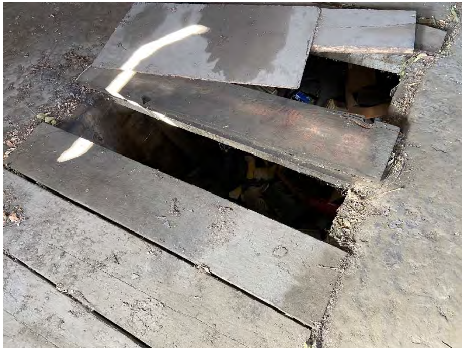
Photograph 24: View of subsurface oil changing pit.
