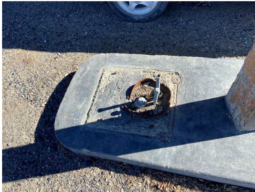
Photograph 4: View fuel island.
