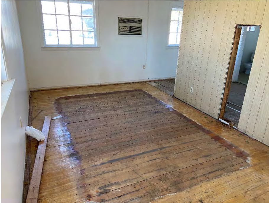
Photograph 7: View of previous motel reception/check in area.
