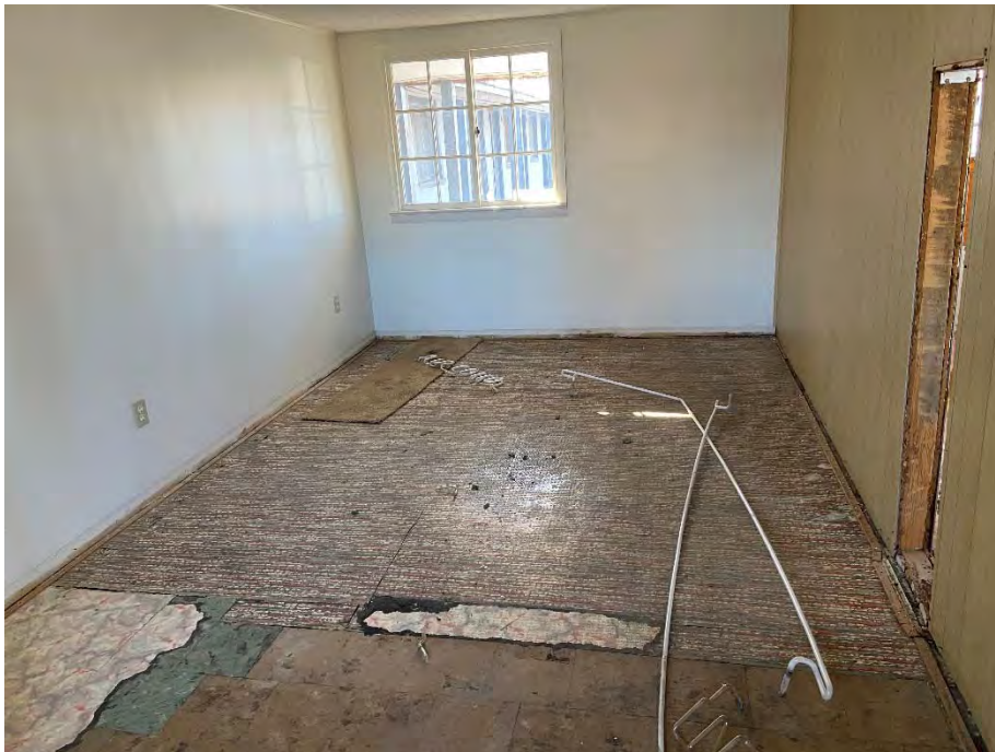
Photograph 8: View of motel room.
