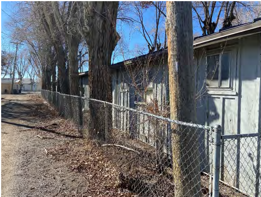
Photograph 6: View of rear portion of the motel building taken facing west.
