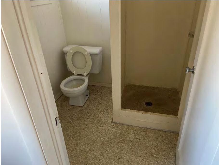
Photograph 9: View of motel room bathroom.
