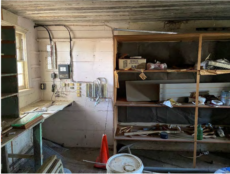
Photograph 11: Additional view of the maintenance area.
