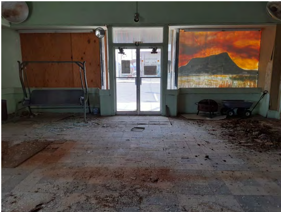
Photograph 4: Storefront as viewed from the interior.
