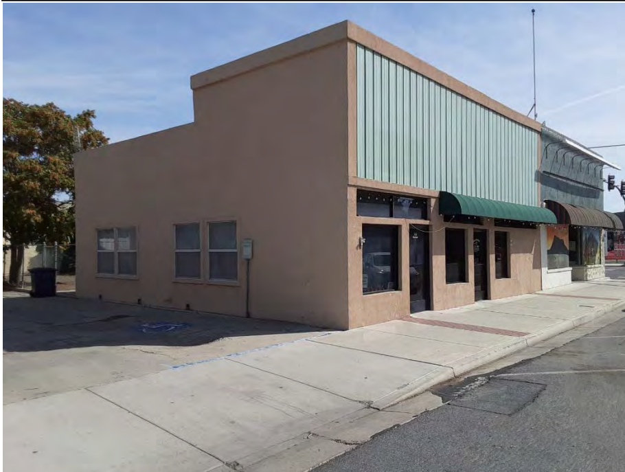
Photograph 10: Adjacent property to the west.
