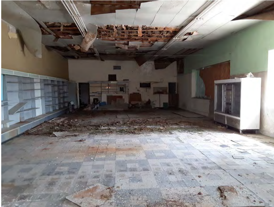
Photograph 3: Interior view of the building.
