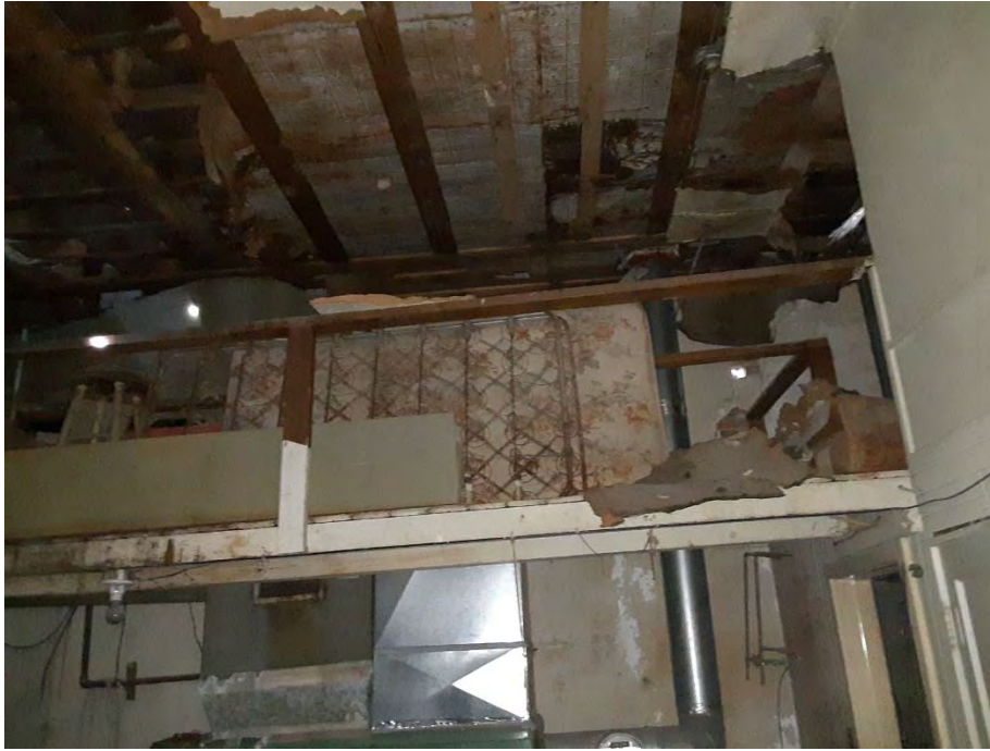
Photograph 7: View of the building ceiling.
