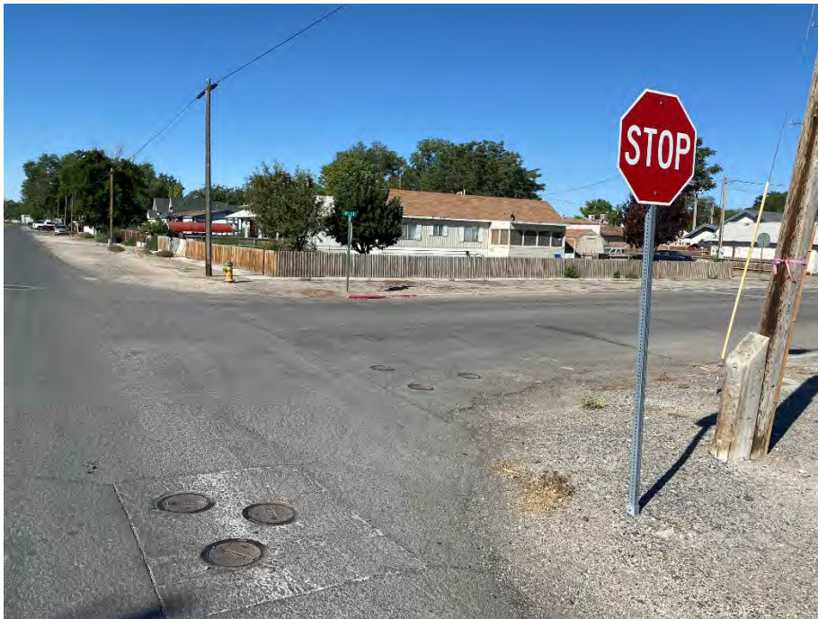
Photograph 6: View of the intersection of 8 th Street and W Broadway, followed by the southern adjoining property.
