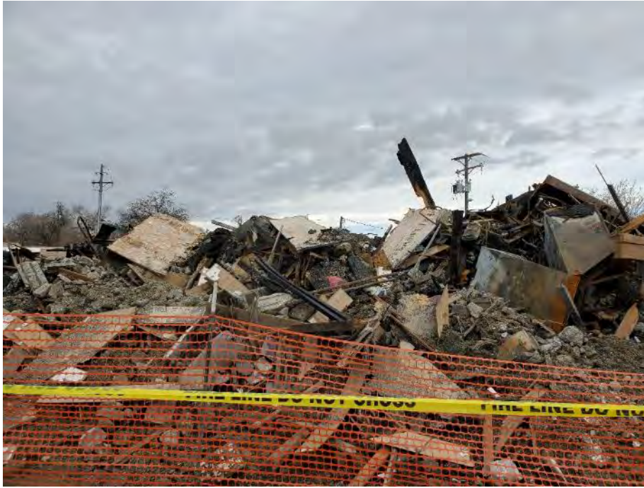
Photograph 3: View of the western adjoining property.
