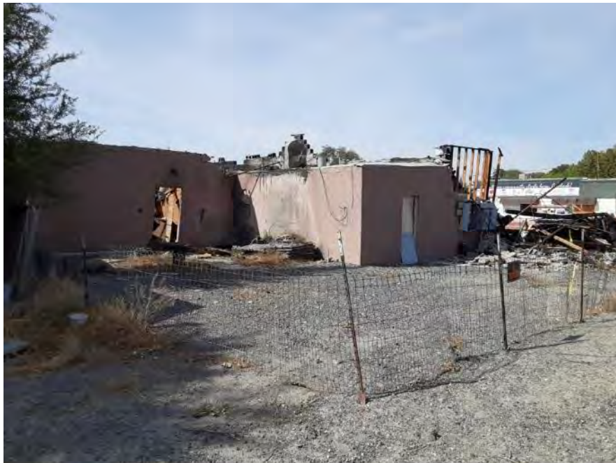
Photograph 6: View of remains of the southern adjoining properties.
