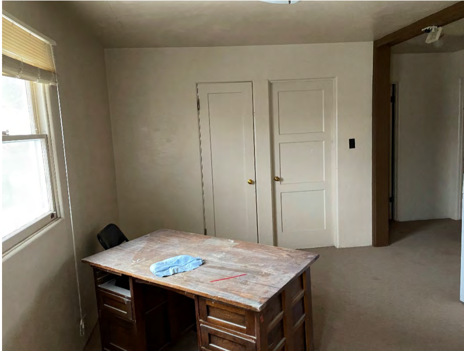
Photograph 7: View of the vacant residential unit.
