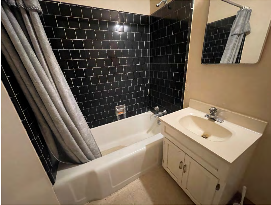
Photograph 13: View of the restroom in the vacant unit.
