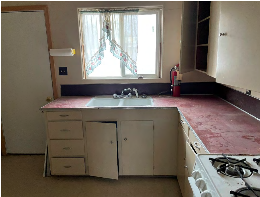
Photograph 8: View of the kitchen area in the vacant unit.
