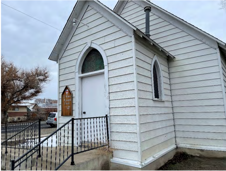
Photograph 1: General view of the Property.
