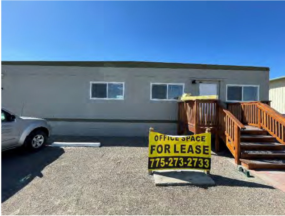
Photograph 1: View of the mobile office building facing north.
