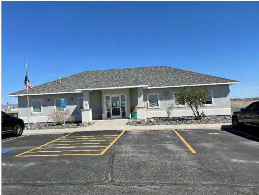
Photograph 24: View of the multi-tenant office building facing south.
