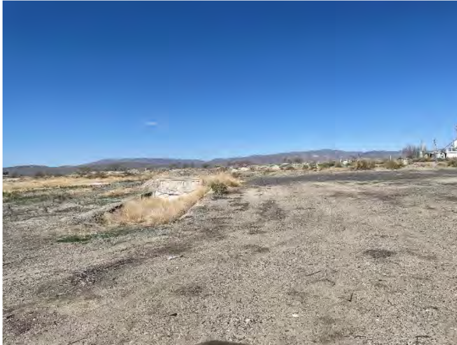
Photograph 21: View of the loading dock located on the northwestern portion of the Property.
