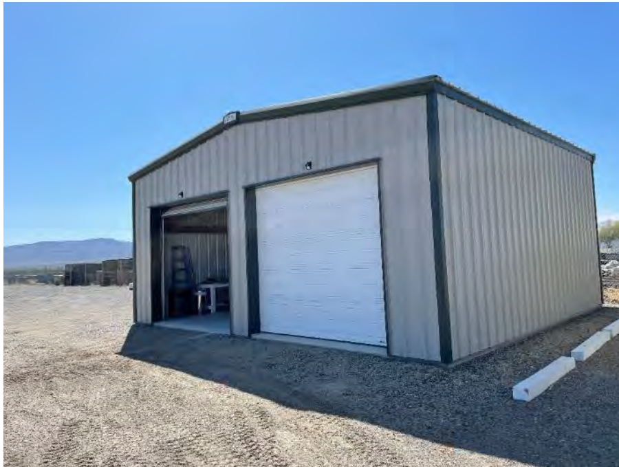
Photograph 18: View of the garage building facing north.
