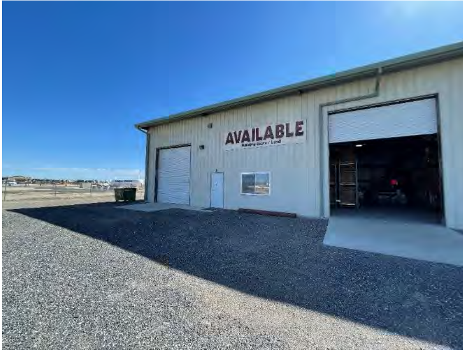
Photograph 5: View of the warehouse building facing west.
