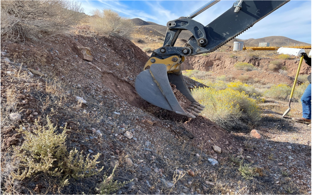
Photograph 3: Sampling of Pile
