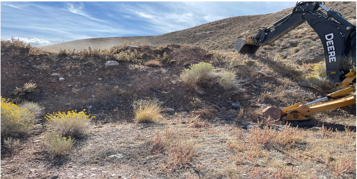
Photograph 4: Sampling of Pile
