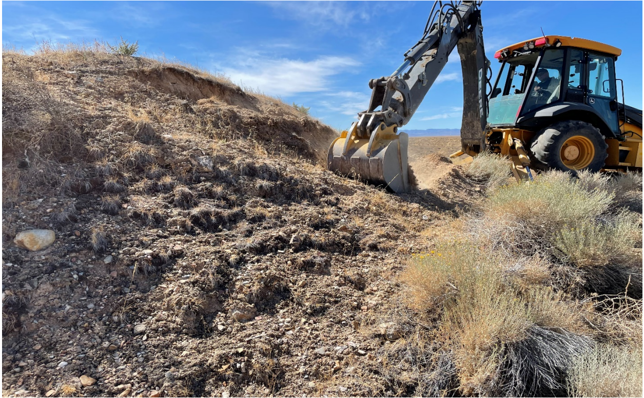
Photograph 5: Sampling of Pile
