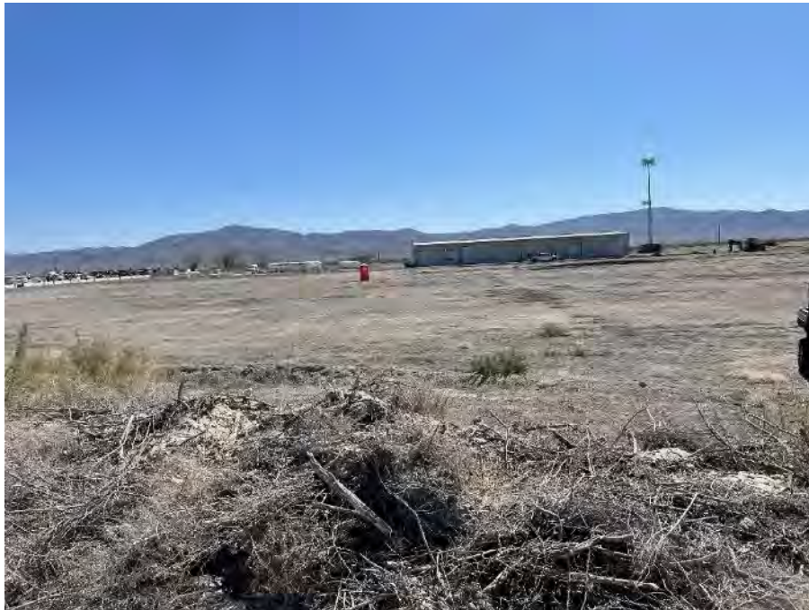
Photograph 20: View of the northwestern portion of the Property with ongoing construction of a new building.
