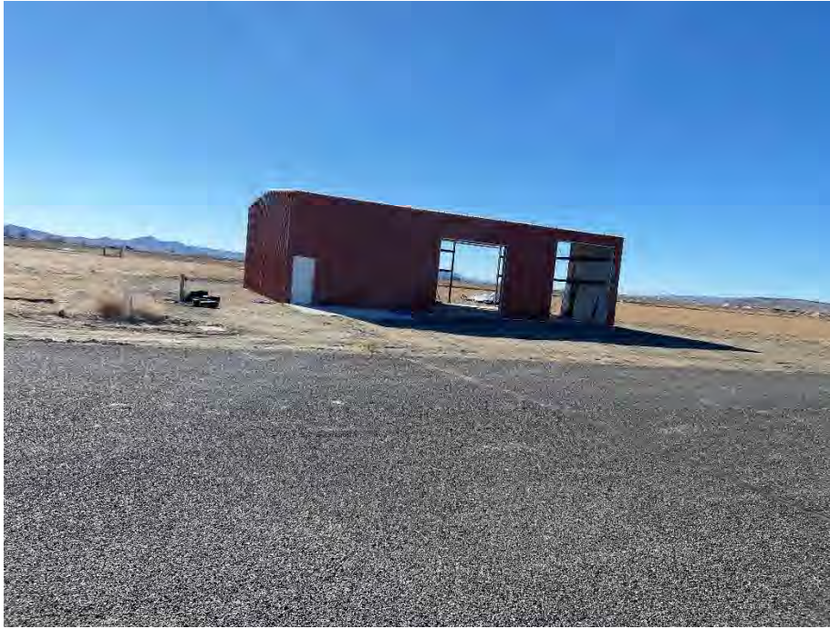
Photograph 3: View of southwestern adjoining property.
