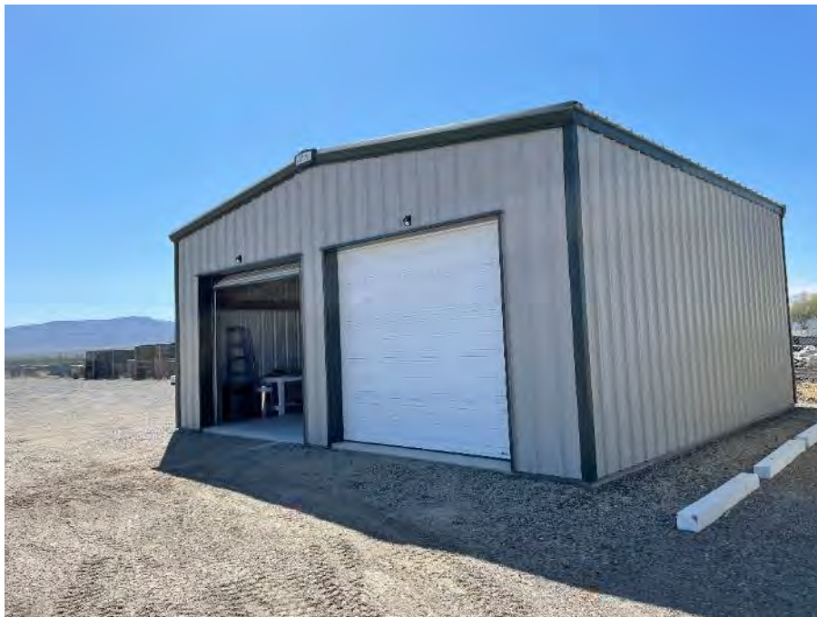
Photograph 18: View of the garage building facing north.
