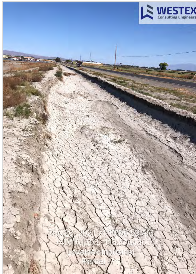
Parcel -71 East side channel facing north
